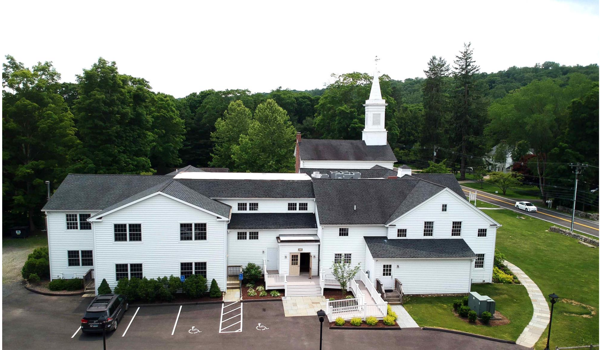
Front View of the Building
