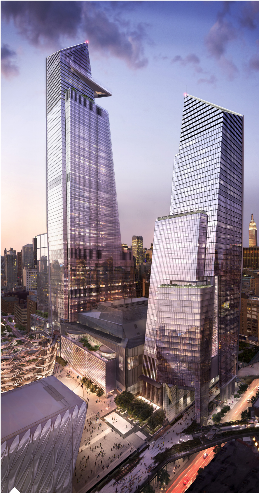
10 AND 30 HUDSON YARDS WITH THE SHOPS AT HUDSON YARDS, LOOKING NORTHEAST
