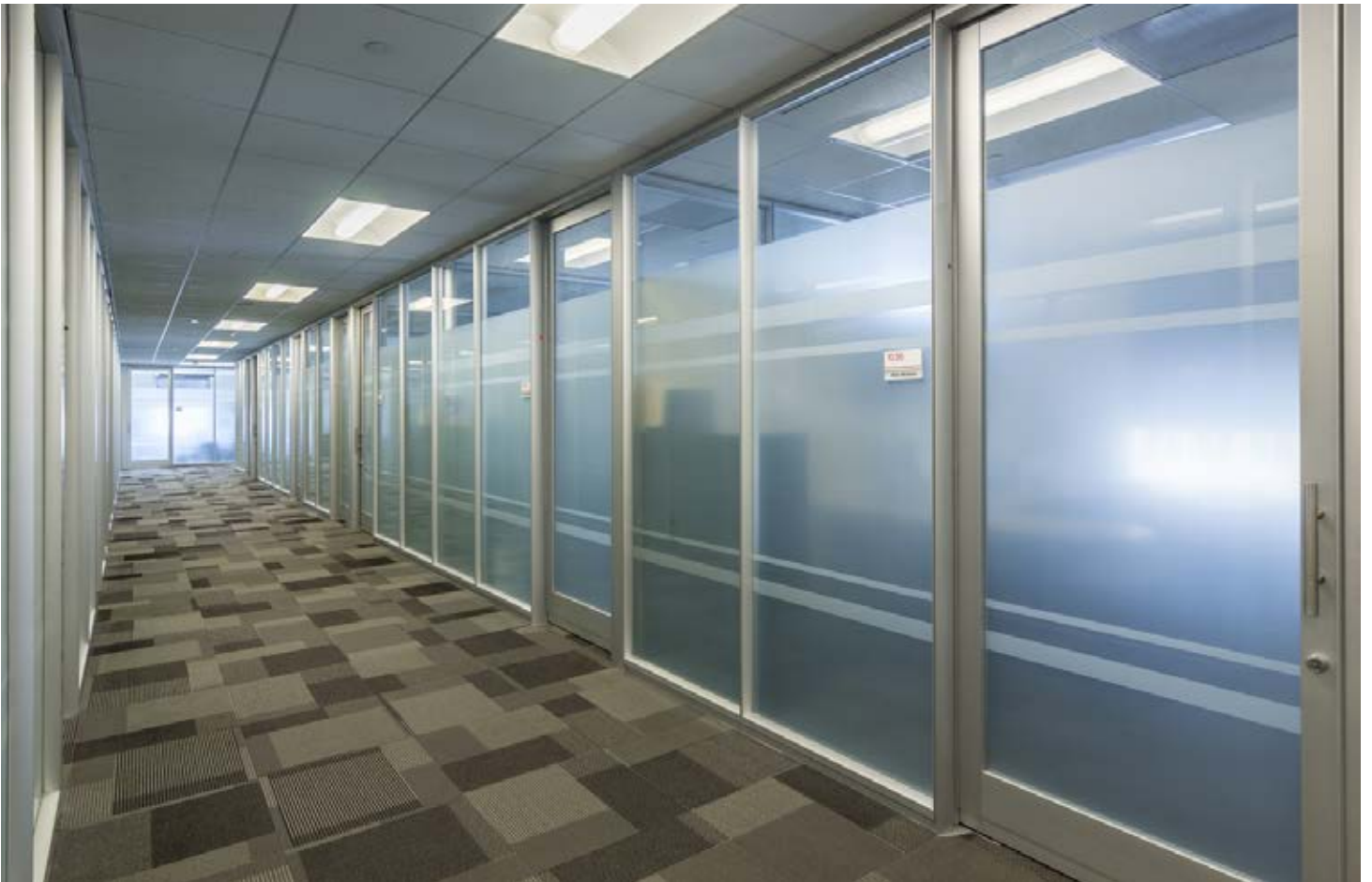
DIRTT wall offices
